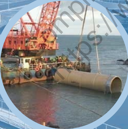
Installation of ocean bed blocks
