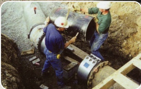
▲ Repair work for pipes replaced underground
