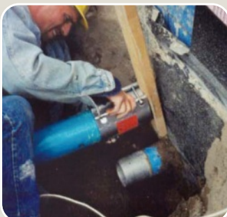
▲ U.S.: sewerage repair work
