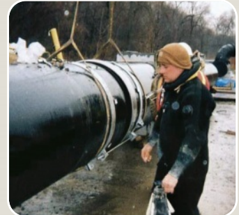
▲ UK: district heating work
