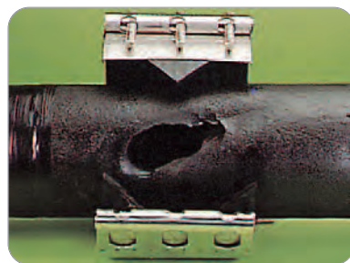
▲ REPAIRING THE PIPES
