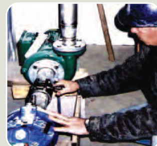
▲ Repair work for high-pressure pump and water supply pipe
