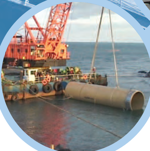
Installation of ocean bed blocks
