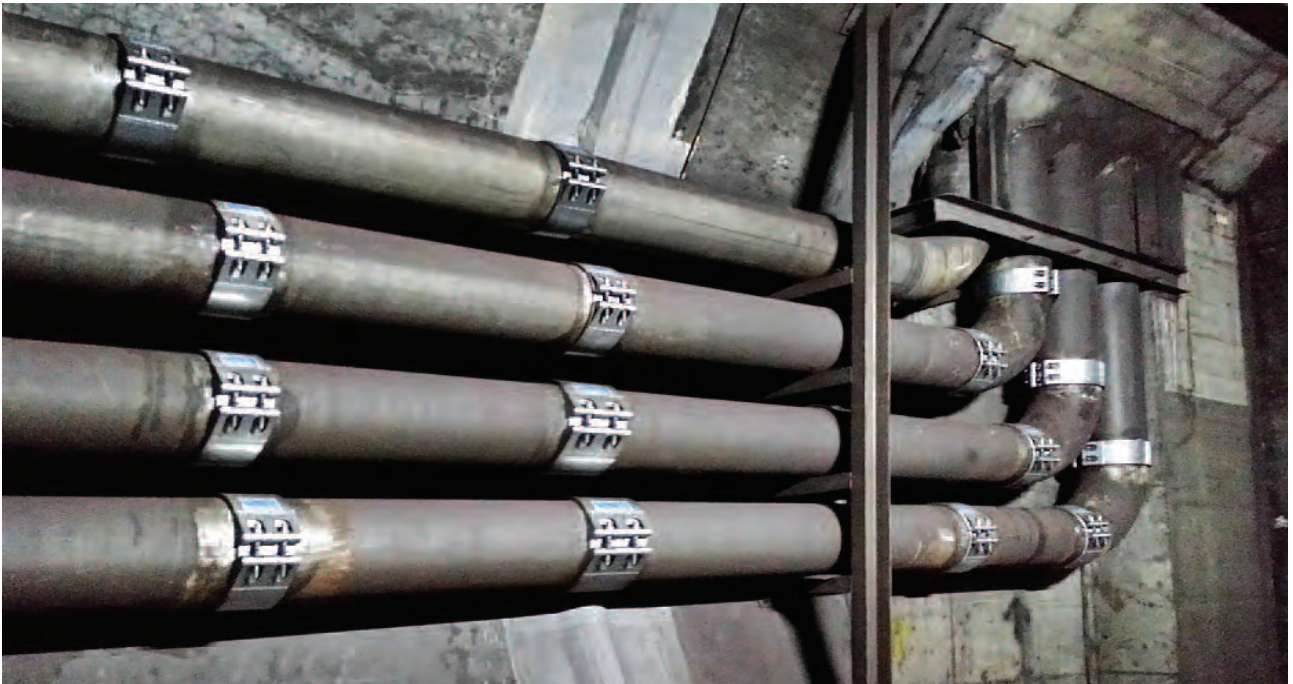
▲ Underground drainage repair(Maintenance) works
