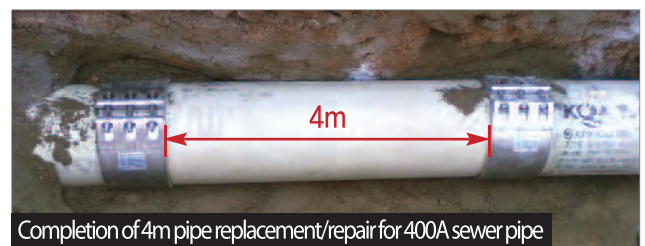
KOWACO sewerage system construction
