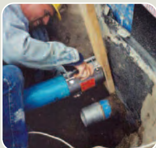
▲ U.S.: sewerage repair work
