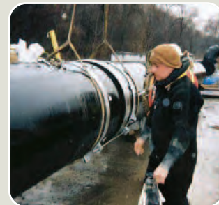
▲ UK: district heating work
