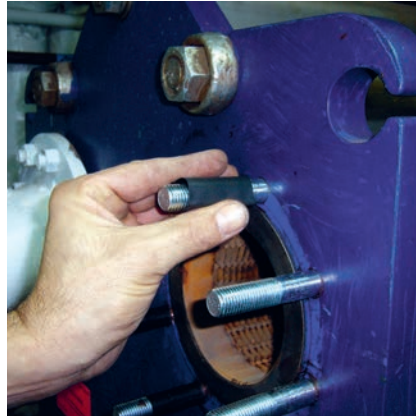
SHUFFLE THE SHRINKING HOSE ABOUT THE BOLT
