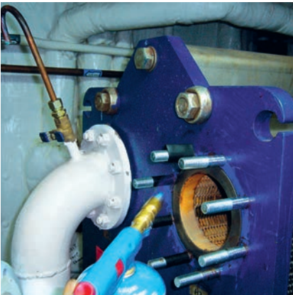
INSTALL THE SEALING
