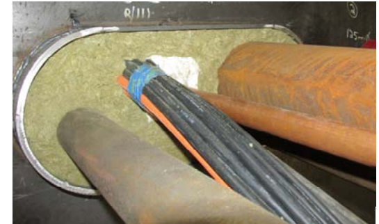
Mineral wool installation
