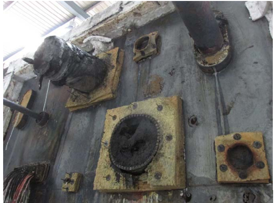
After a fire test
